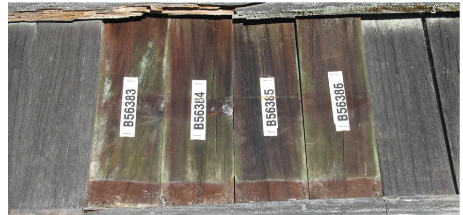
Flat panels Vulcan Radiata 230°C after 11 years exposure, Rotorua.
