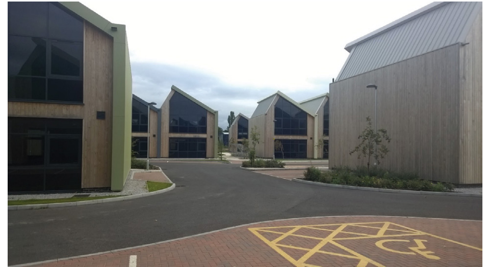
Vulcan Flatsawn Cladding commercial development Robin Hood Airport, UK. Installed 2016..
