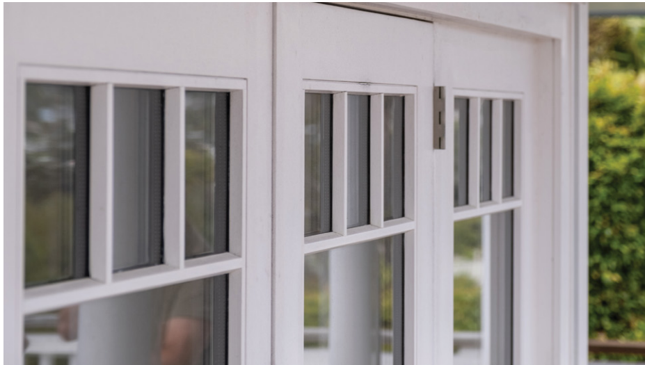
Vulcan window joinery Whangaparoa, New Zealand. Installed 2010.
